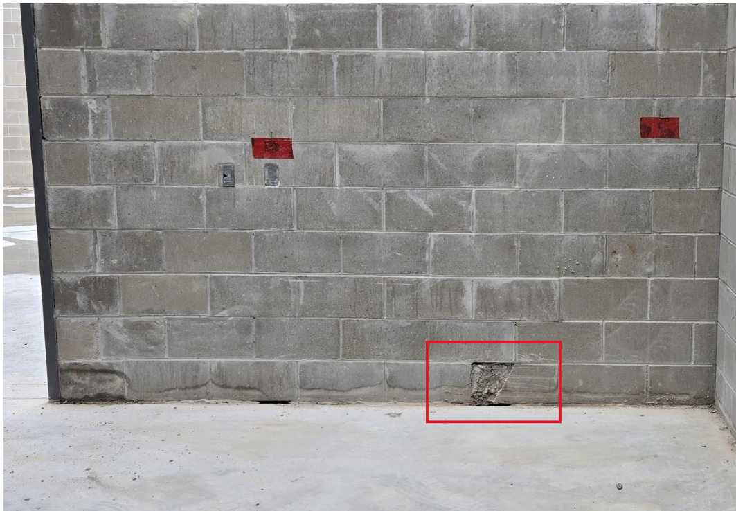
14. Area 2A - Damaged CMU block
