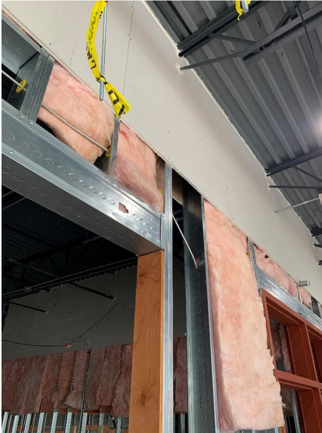
8. Area 5 – Stud framing and wall blocking installation in progress
