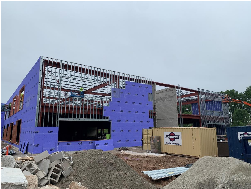
12. Area 4 – Exterior metal stud framing, sheathing, and window framing installation in progress
