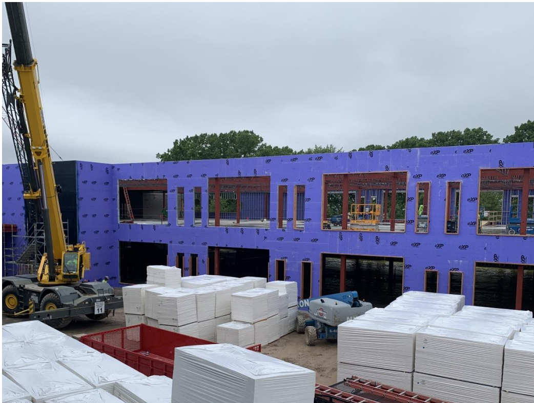
10. Area 4 – Exterior sheathing and wood framing installation in progress
