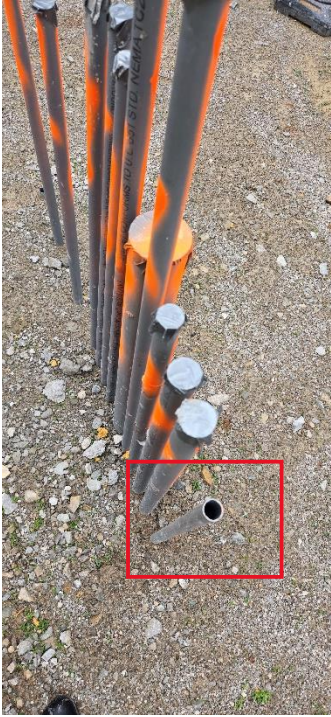
16. Area 6 - Damaged metal stud
