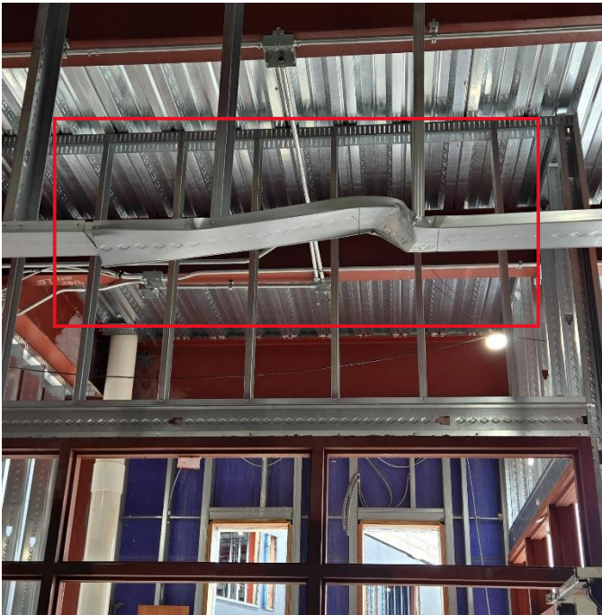
16. Area 6 - Damaged metal stud
