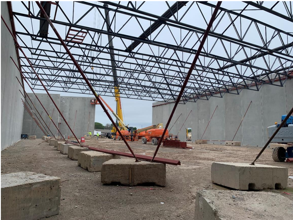
2. Area 6 – Precast back up panel and gym roof structure installation in progress
