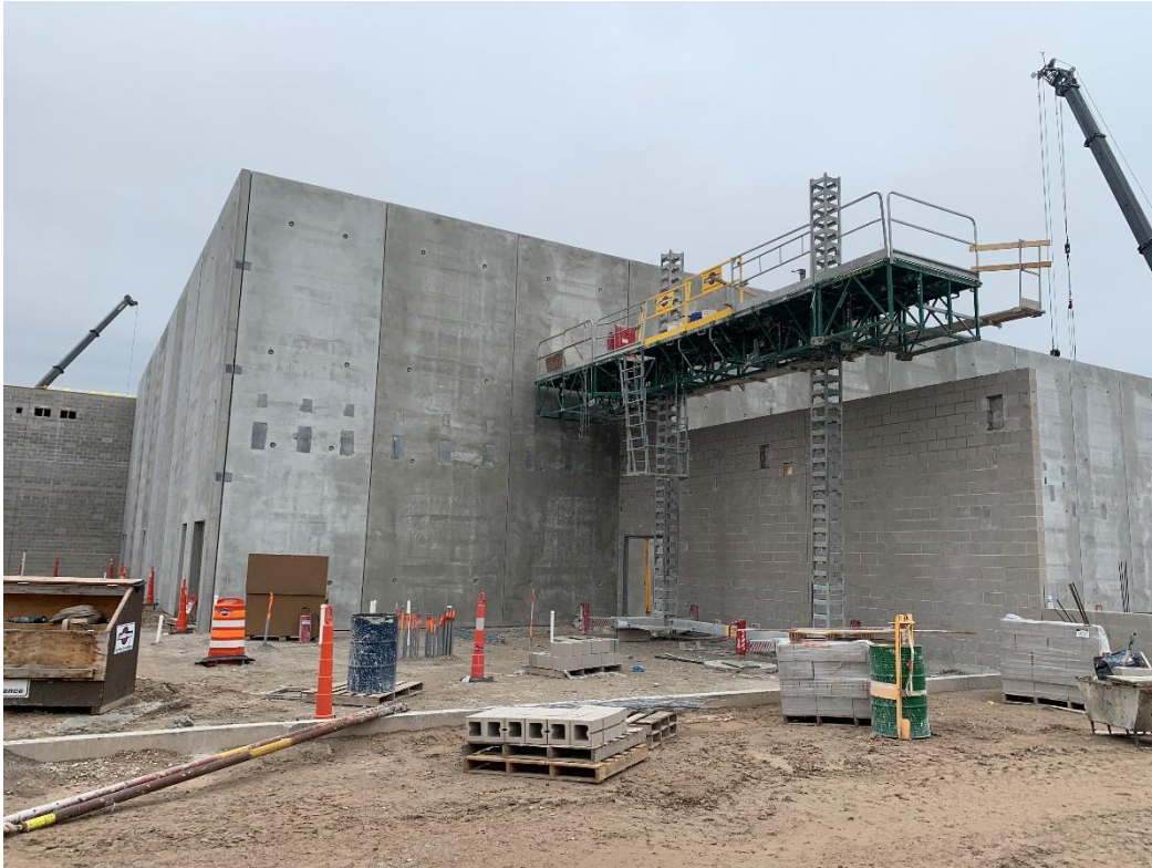
2. Area 6 – Precast back up panel and gym roof structure installation in progress
